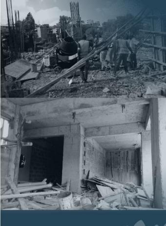
Casting of parking level columns ongoing in preparation for casting.of wing 02 of ground floor 01.
