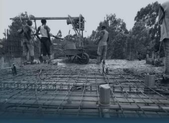
Constructon work for the ground floor slab formwork + support in preparation for eventual casting.
