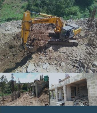
Backfilling at the parking level in preparation for casting the second wing of lower ground slab. De-shuttering of formwork plus walling on lower ground level
