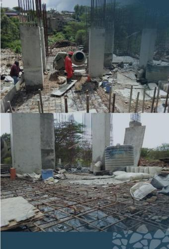
Casting of lower ground slab after column erection. This overlap of activities allows for time to complete necessary foundation works and parking level without losing time on the project.
