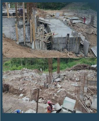
Completion of all foundation bases, ground beams, columns, lift core foundation as well as 100 CM underground water tank.
