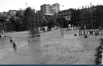
Ground floor slab cast. Now onto the ground floor columns in preparation for the first floor slab.
