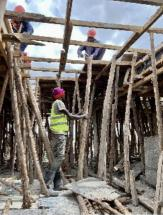
> 9th floor slab shuttering ongoing in wing B in preparation for steel fixing.
